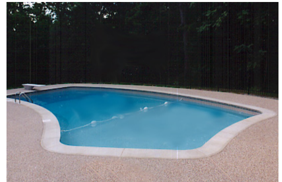
After installing the liner and filling with water, the finished pool!
