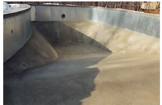
A typical vermiculite pool bottom just before the liner is installed.
